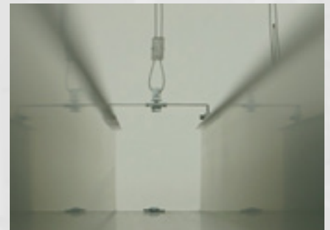
Image displaying adapter and wire suspension in-situ, offering a mechanical fix to the services which are secure and level.
